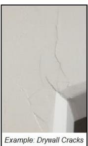
**Note:** Occasionally a problem called "truss lift" occurs, causing a slight buckling of the ceiling drywall during cold weather. Truss lift lasting more than one winter may be a permanent feature of the truss design (vaulted ceilings are more susceptible to this). Keep in mind that texture can appear inconsistent.
