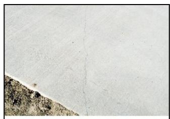
The photo above is an example of a hairline crack, which is not covered, unless the opening is wider than 1/4"
