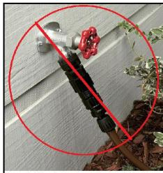
Example: Pipes that are frozen due to not detaching hose from the outside faucet will not be covered under the Builder's Warranty.
